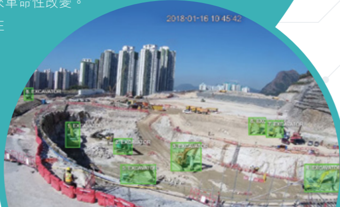
項目可同時追蹤及監察到8部挖土機。 The technology can be used to monitor the operation of up to eight excavators at the same time.
