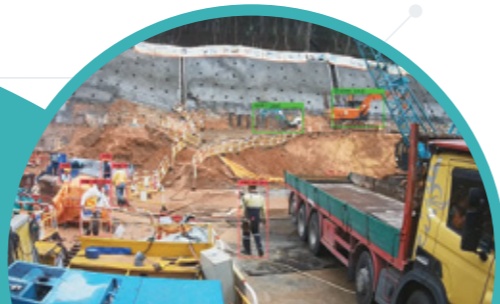
在俊和建築工地使用先進的電腦視覺算法，追蹤建築工人和挖土機的狀況。 Advanced computer vision algorithms are used to track worker status and excavator use at Chun Wo's construction site.
