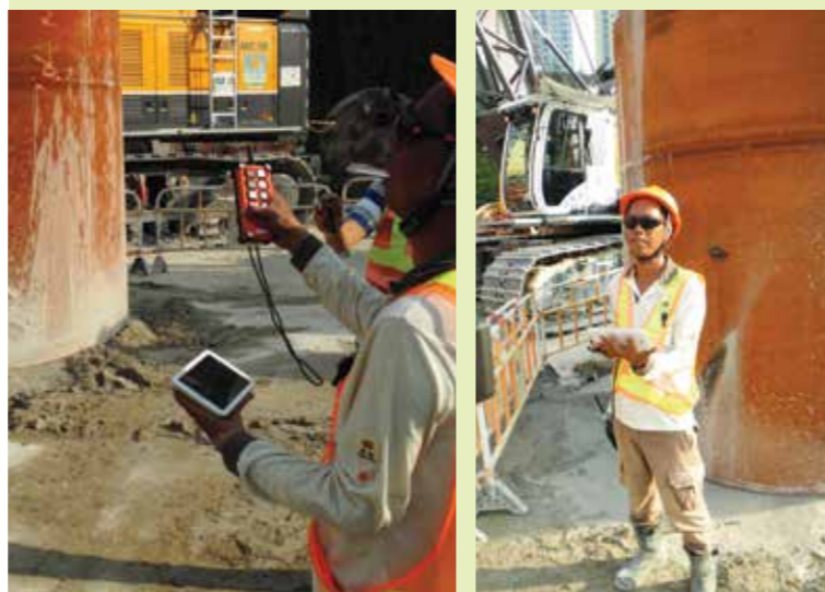
遙控混凝土載斗配備電子控制箱和視像鏡頭，在地面的工友可控制和透過平板電腦監視傾倒混凝土的情況。 Through remote control and a web cam, the Unpiloted Concrete Skip enables workers to control and monitor the operation through a tablet, thus all necessary operating procedures can be done safely on the ground.
