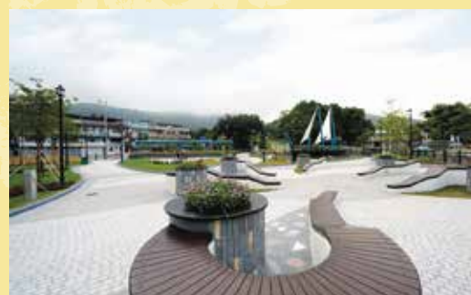
西貢福民路明渠改善計劃，是首次以「新工程合約」形式運作並由俊和承建的工程，改成箱形暗渠後的上蓋成為福民花園。 "Improvement of Fuk Man Road Nullah in Sai Kung" is the first project which adopted NEC mode of operation and constructed by Chun Wo. The Nullah was rebuilt into a box culvert and Fuk Man Park was built on it.
