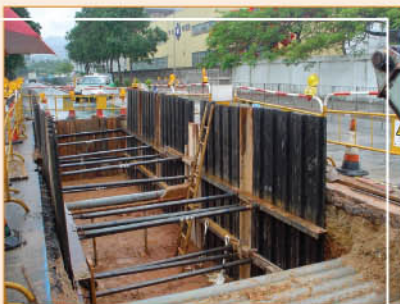
明坑開挖及臨時支撐。 Open trench excavation and shoring installation.
