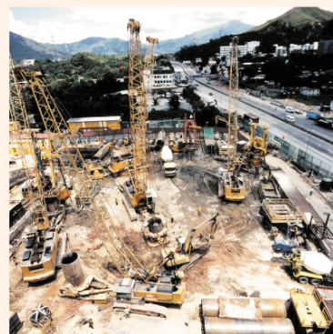
博愛醫院重建項目地盤開拓及地基工程 Site formation and foundation works for redevelopment of Pok Oi Hospital
