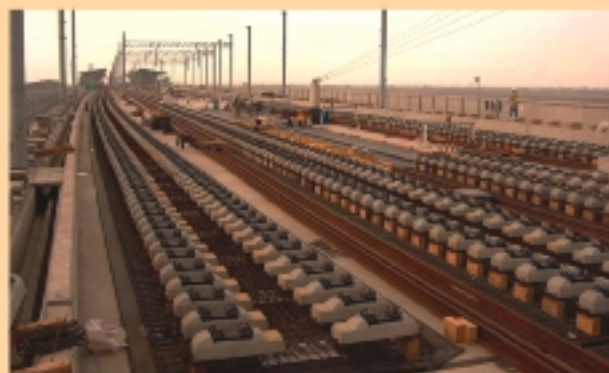
日間軌道調較工作。 Track setup and adjustment at daytime.
